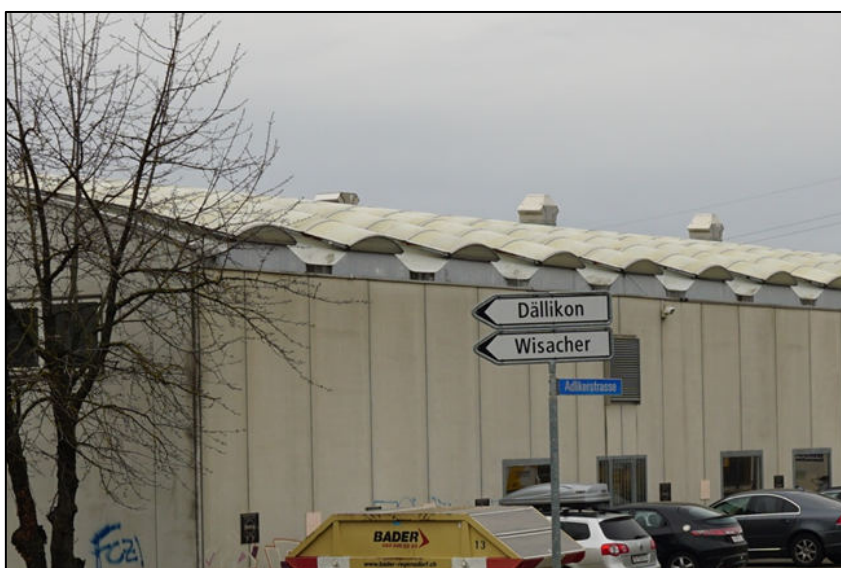
Detail Dachrand Halle
